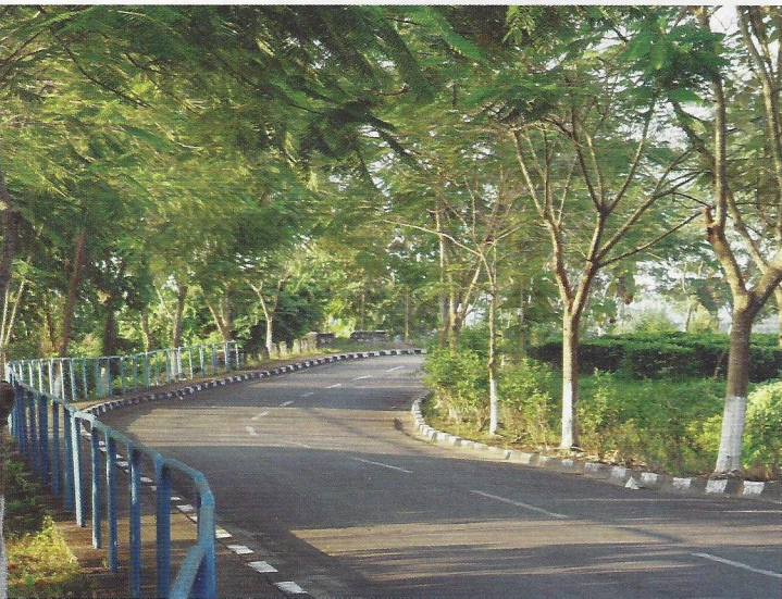
APPROACH ROAD TO THE SCHOOL COMPLEX
